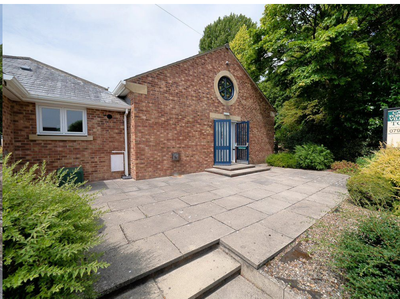
Doors from Main Hall leading to Patio
