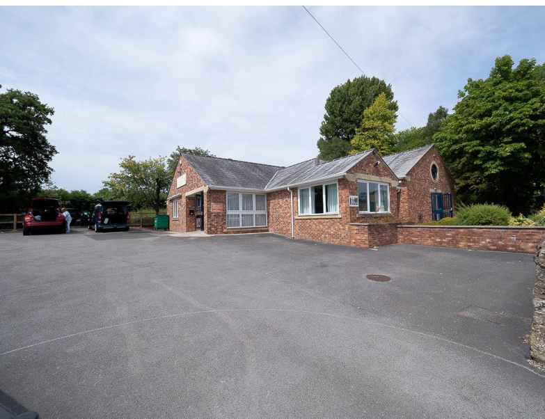
Calcutt Village Hall showing Car Park
